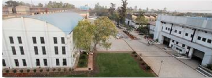
UNIT-1 CAST PRODUCTS PLANT BUILT UP AREA: 125,000 SQ. FT.
