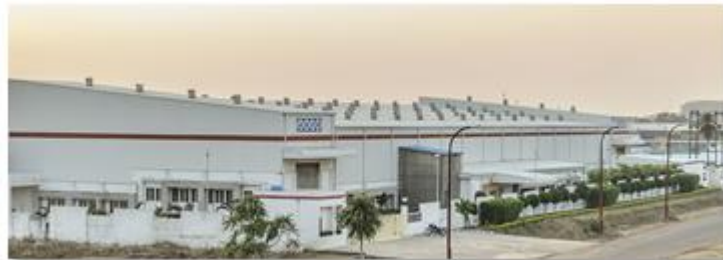
UNIT-3 SEZ PLANT BUILT UP AREA: 50,000 SQ. FT.
