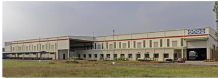
UNIT-2 FABRICATED PRODUCTS PLANT BUILT UP AREA: 155,000 SQ. FT.
