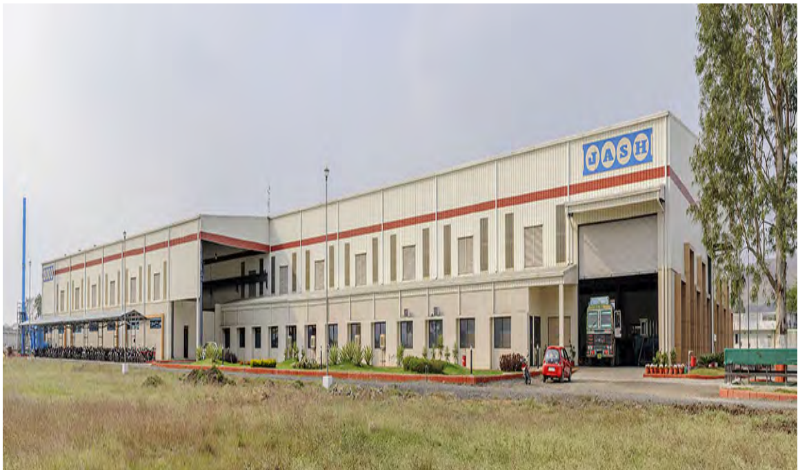
Fabricated Products Plant II: Bardari, Indore
