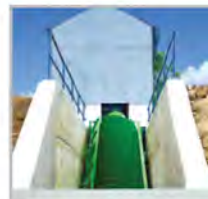
Archimedean Screw Turbine
