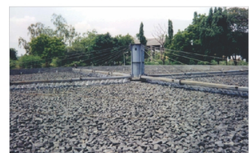
Trickling Filter
