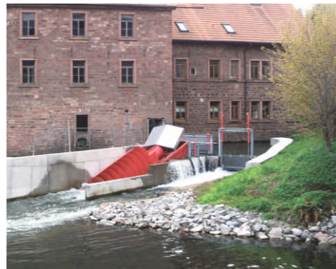
17.4 kW System, Lohram Main
