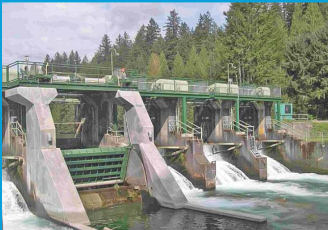
6000 x 2400 mm, Crest Gates, Landsburg Fish Passage Ravensdale, WA, USA
