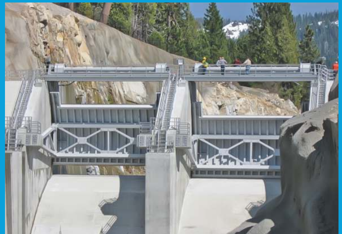
10950 x 5650 mm Tainter Gates L.L. Anderson Dam. CA, USA
