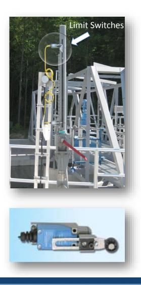
Remote indications of gate opening arrangement is provided on rising spindle gates to indicate "OPEN" or "CLOSE" position of gate at remote position in control room.
