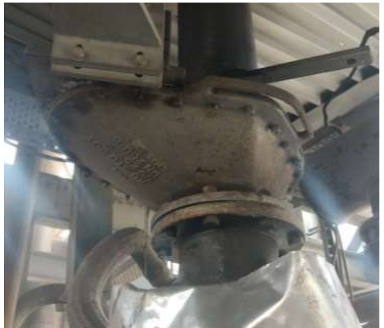
KU-HT DN200 Installed at M/s J.K. Cement Ltd.
