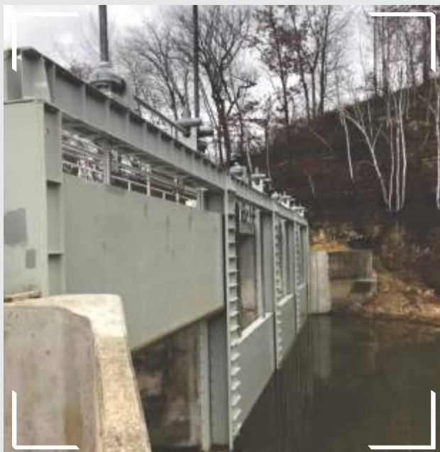
Hillsboro Dam, WI, USA Structural Steel Roller Gates 20' X 6.75' - 4 nos.
