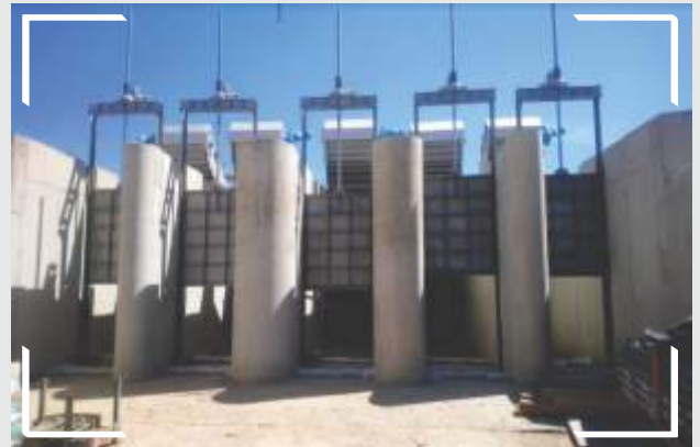
Daldowie WWTW, UK. Side Wall Embedded Open Channel penstock 1600 x 1900 mm - 10 nos.
