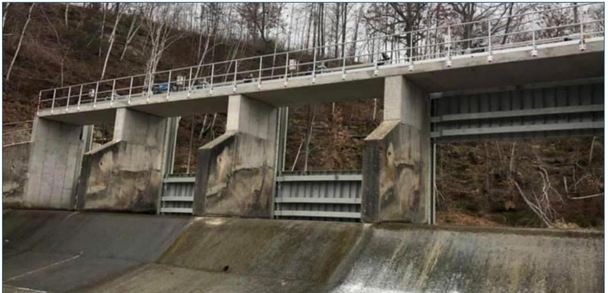
240" x 81" Structural Steel Roller Gate for Hillsboro Dam, UT, USA
