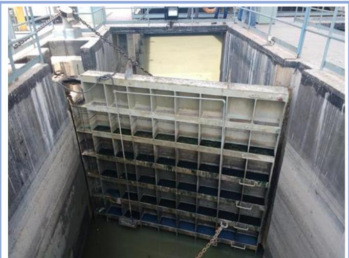
147.6” x 204.7” Structural Steel Miter Gate for Britannia outfall
